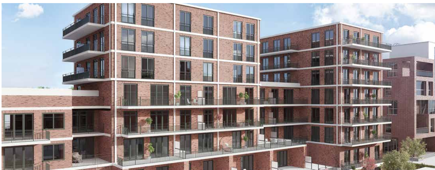
Amstelkwartier, Amsterdam | Project under construction
