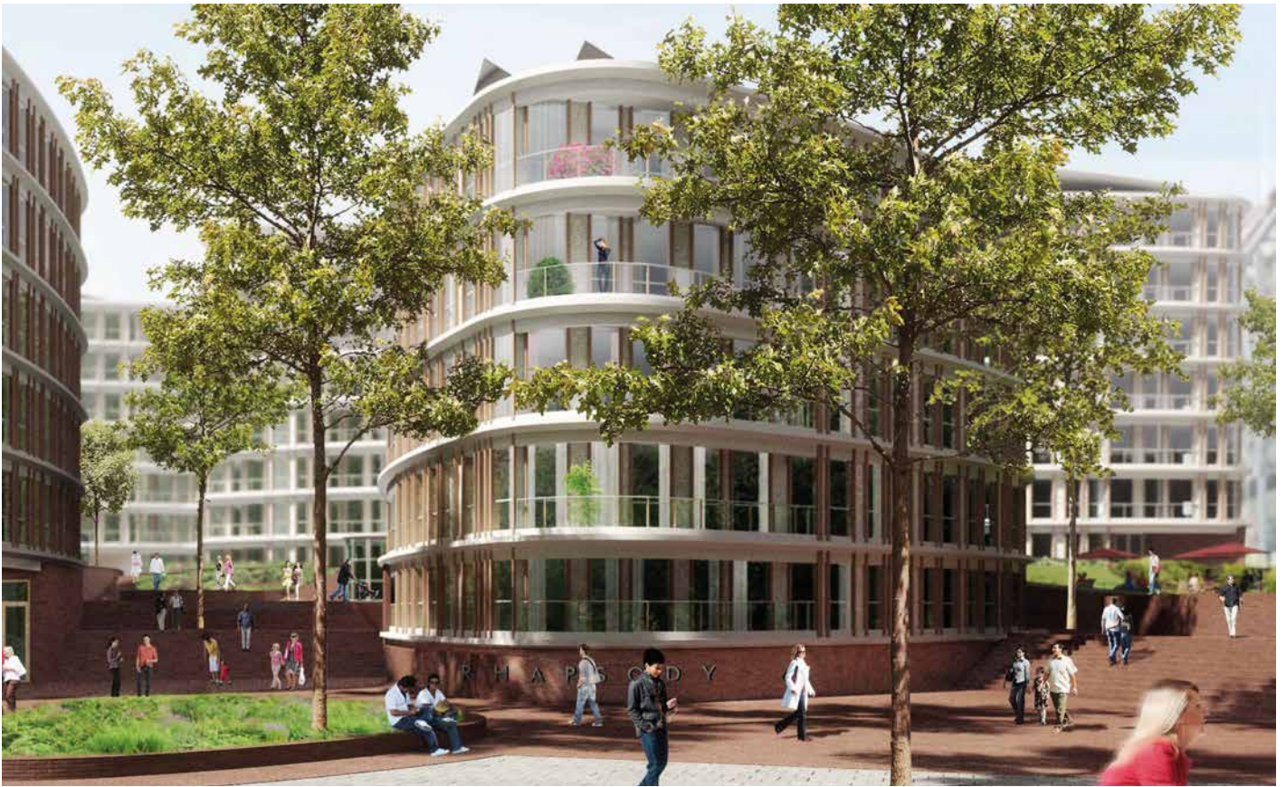
Rhapsody, Amsterdam | Project under construction
