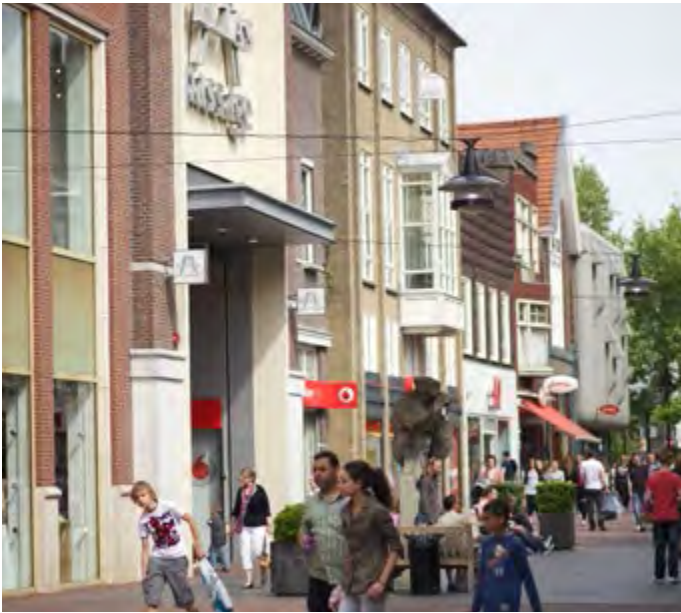
Elzaspassage, Helmond | Energy label C | BREEAM Good asset and Very good for Management; improvement of management score
