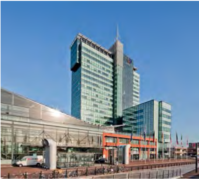
UP Building, Amsterdam | Energy label A
